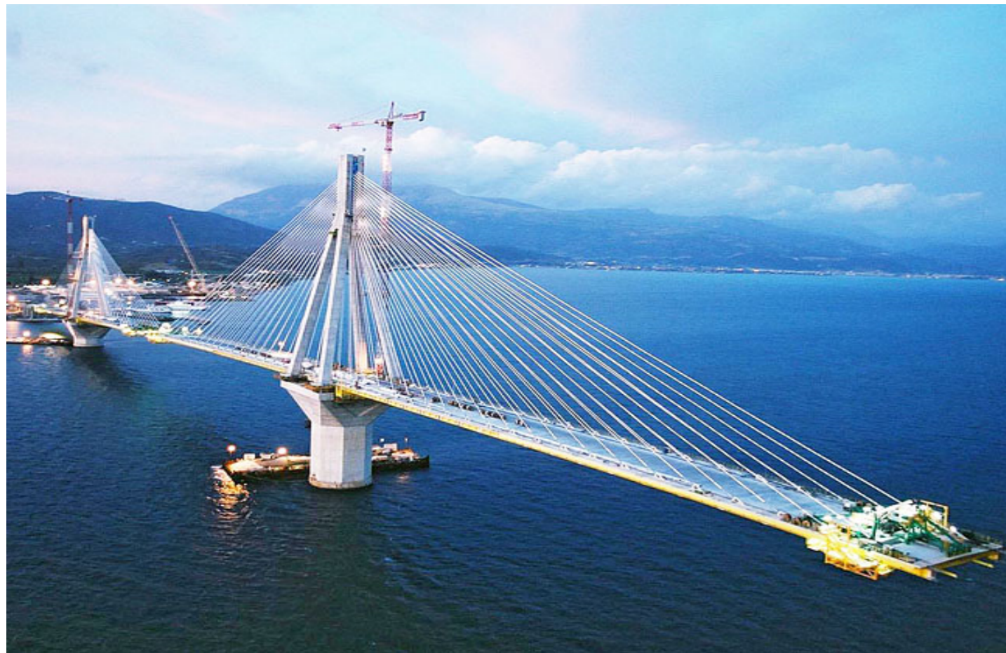
Above. Full view of the bridge.
